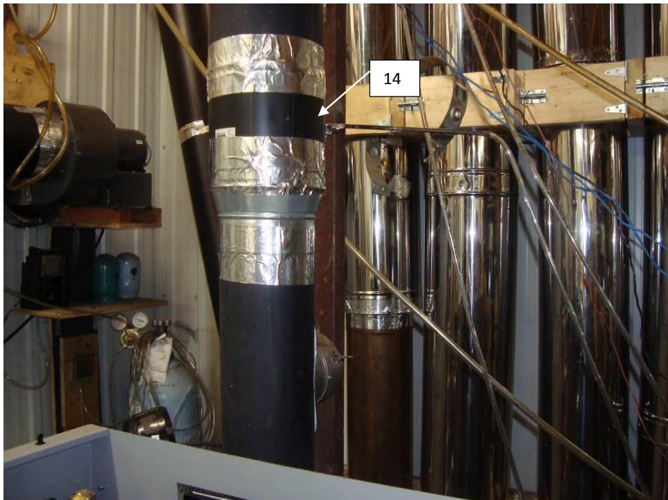
14 : Draft sampling port located 6 in.from the flue outlet
